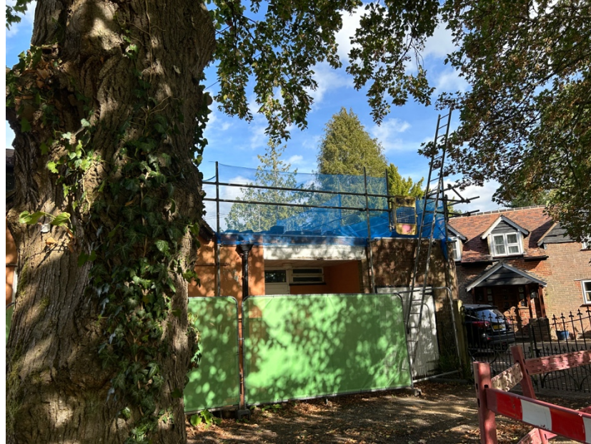
LEFT - removal of tiles from Hall roof
