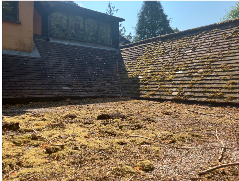
LEFT - Exposed former hall floor
