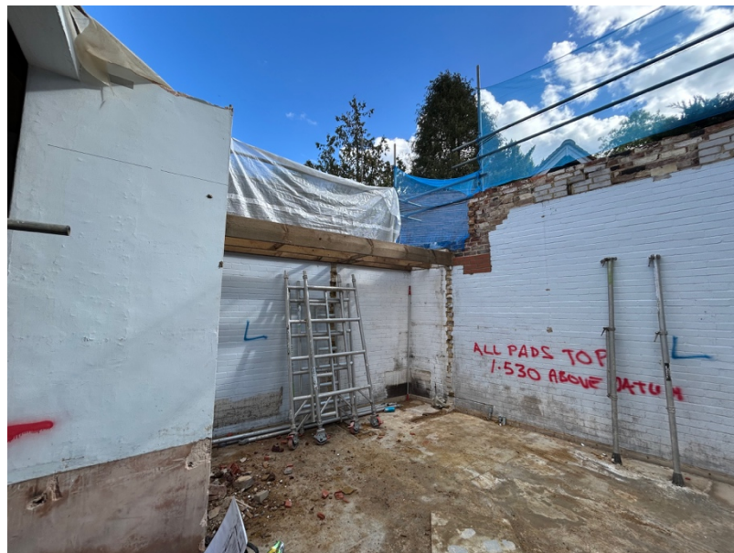
Left: view through hall, post-demolition, rear to front
