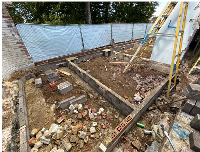
Left: new wall construction in progress
