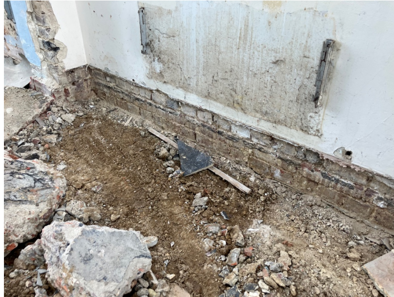
Left: demolition in progress
