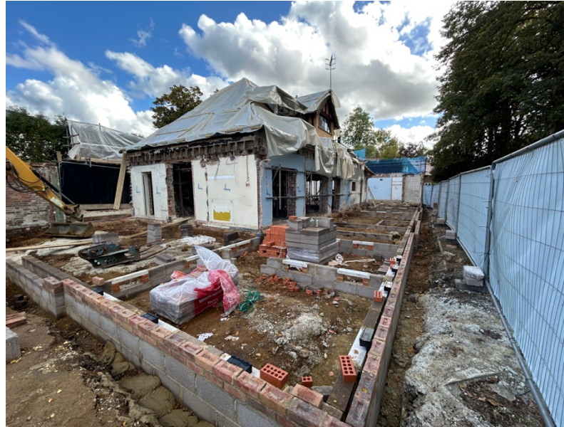
Left: new foundations laid and groundwork commenced
