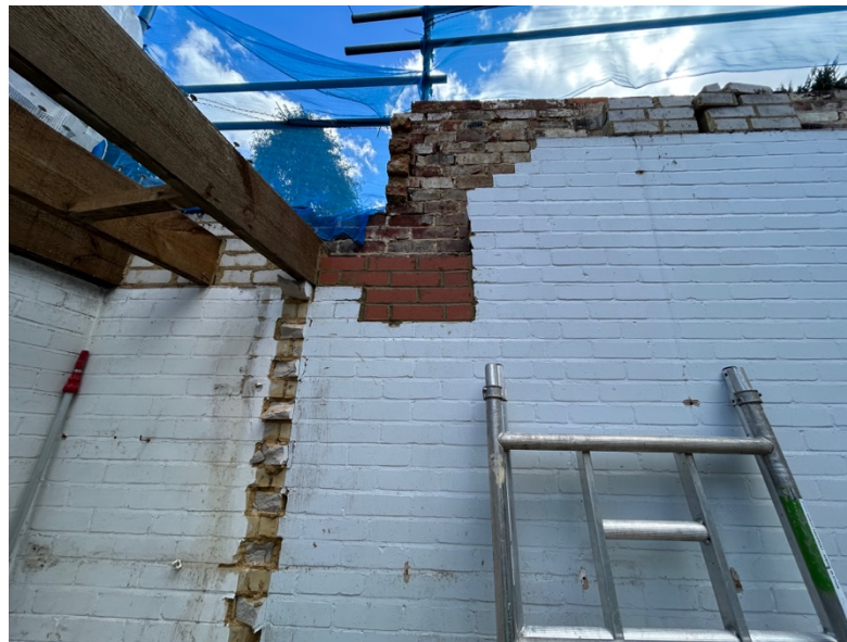
Left: engineering bricks installed at rear of hall to receive new RSJ
