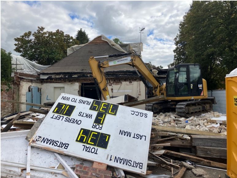
Left: Site view showing only core hall remaining post demolition work
