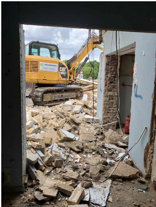
Left: demolition in progress – internal view
